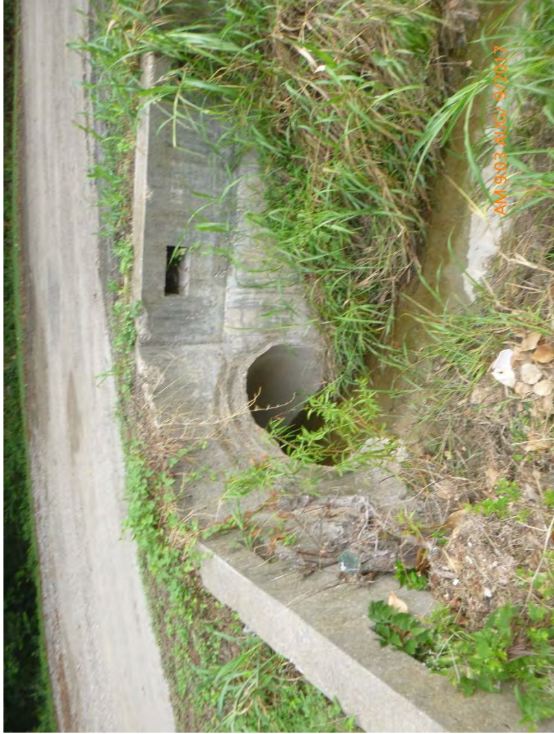
Photo 2. View, facing northeast, of culvert draining to Crossing 1.
